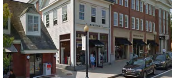
Storefronts turning the corner to enliven mews
