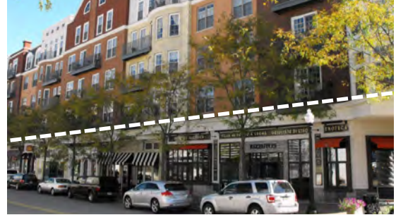
Ground floor storefront continuity
